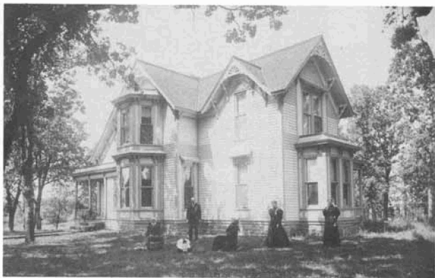
Pictured is the home built by Lemuel Potter and now owned by Dinsmore Brandmill, a grandson of the Potters. Built in 1886, it was damaged considerably by the tornado in 1968, repaired, and occupied by the Brandmills. This is a century farm. Identified in picture left to right: Lemuel Potter, Parke Brandmill, Charles Brandmill, Honoria Potter, Elma Potter Brandmill, and Nora Potter Sisco.
