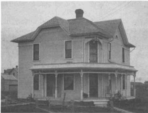
The J. W. Conway house, built in 1897 on the east side of Elma. In the background to the extreme right is the blacksmith shop and to the left of the blacksmith shop is the wagon shop that served Elma when the town was much younger. James and Loretta Stapleton made their home here for years; it is now occupied by the Kimbles.
