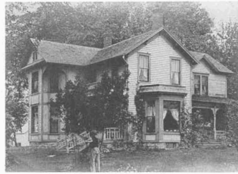
The Truman Robison house, also known to many as the "Burgess House" and the "Knippling House" as the years went by, is now owned by Pat Fogarty who was occupying the house when it was virtually destroyed by fire two years ago.
