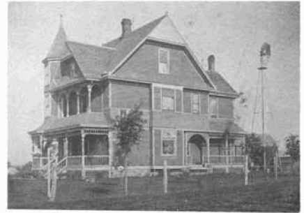
"Grand View Elma," the William Watson house until September, 1908, was moved to the site where Emma Havlik's house is now. Frank Elwood and a Parker family lived there until it was torn down in the 1930s.
